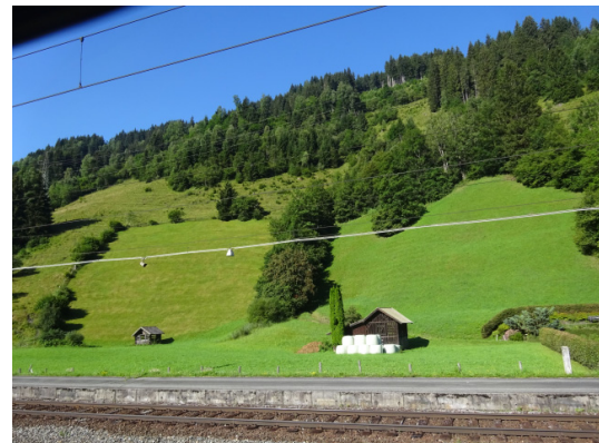
Figure 3c. This energy landscape in Carinthian Mölltal in Austria shows different layers of energy production and impact on the landscape. Foreground: electric train line and electricity high voltage cables. Middle: agriculture including modern hay balls; background, forestry. These very intensive and close layers are dominating the Alpine valleys in Austria. (Photo: Alexandra Kruse 2016)
