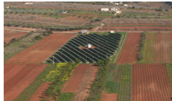
Figure 30b. PV-Panels in parallel to the airstrip of Athens Airport. This can be considered as best practice as the installation respect at best the already given rectangular layout of infrastructure and agriculture. (Photos: Alexandra Kruse 2017)
