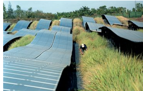
Figure 25d. Type b) Agrinerie® (2.1 MWp), La Reunion (FR). It combines energy generation from PV and lemon grass production. This dual land use design pattern enabled the developers to get the approval for the realization of a system, since in French overseas islands it is not allowed to build on ground PV, because of land and landscape protection rules. (Photo: Akuo Energy)
