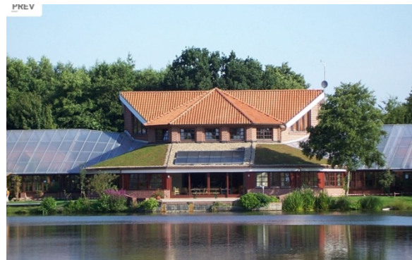
Figure 34b. Historic-Ecological Education Center Papanburg/Germany, built in 1988: Towards the North there are earth walls as energetic protection, towards the south a winter garden, which serves as semi-tropical greenhouse and as corridor between the accommodation units and common facilities. The bricks which store the temperature have been recycled. (Photo: http43 )
