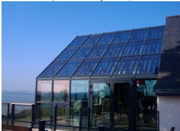
Figure 25b. Type a) Roof integrated photovoltaics. Glass-glass PV modules can be used in replacement of standard glazed surfaces (facades, roofs, skylights) in building's envelopes, coupled with standard framing systems. (Photo: courtesy of Ertex Solar)
