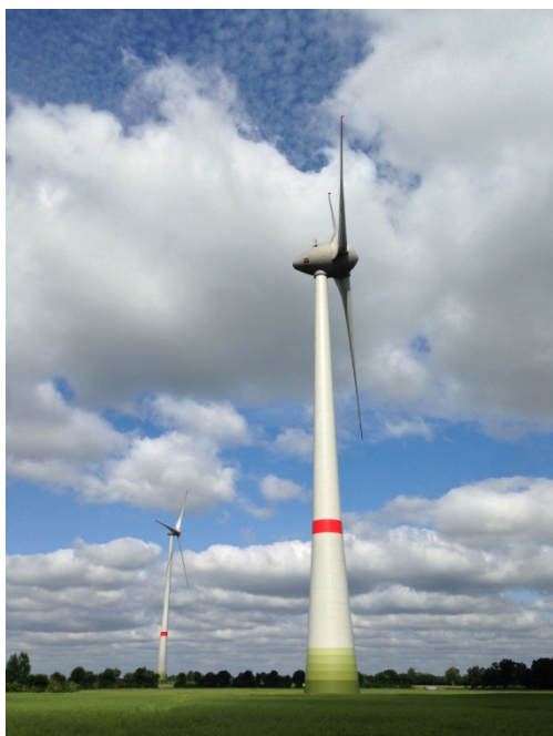
Figure 29a. Onshore wind farm near Diepholz, Germany, with the currently world's highest performing onshore wind turbine, i.e. the Enercon-126, with a hub height of 135m (443 ft), rotor diameter of 126m (413 ft) (Photo: Olaf Schroth 2015)
