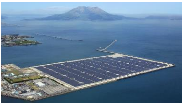
Figure 30a. The ‘Floating’ solar power plant in Kagoshima Bay, Japan can be considered as a good example for saving space. The panels over water have a cooler temperature which makes them more efficient. Finally the blue colour of the panels matches with the blue of the water, hence the panels do not disturb aesthetically. (Photo: © KYOCERA Corporation)
