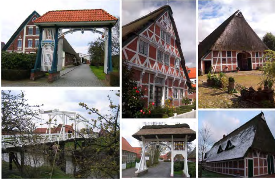
Figure 6: The Altländer Farm is a special type of Northern German half-timber hall house with mixed use. Dominating colors are red and white. Most of the 300 – 400 years old buildings are protected monuments. The Hogendielsbridge is a reconstruction, recalling the Dutch heritage. Still 12 original parade gates exist insitu. They are known only from the Altes Land. (All photos by Kruse, A.)
