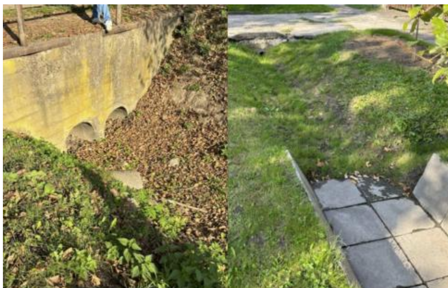
Figure 4. Examples of the problems in the Ördög Ditch: on the left is the dry upper section, on the right the sediment-filled bed (Source: Júlia Anna Sebestyén, 2023)
