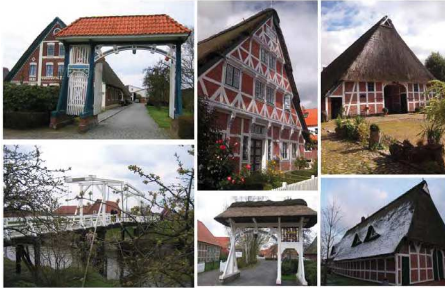
Figure 6: The Altländer Farm is a special type of Northern German half-timber hall house with mixed use. Dominating colors are red and white. Most of the 300 – 400 years old buildings are protected monuments. The Hogendielsbridge is a reconstruction, recalling the Dutch heritage. Still 12 original parade gates exist insitu. They are known only from the Altes Land. (All photos by Kruse, A.)
