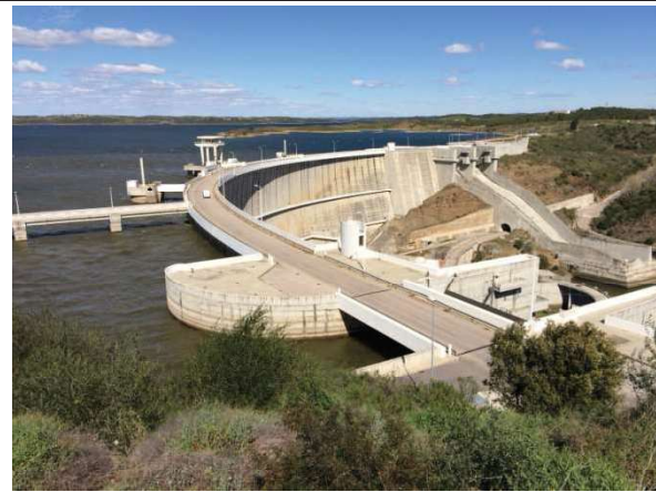
Figure 23b. Large hydro power plant Alqueva II in Portugal (Photo: Naja Marot 2015)
