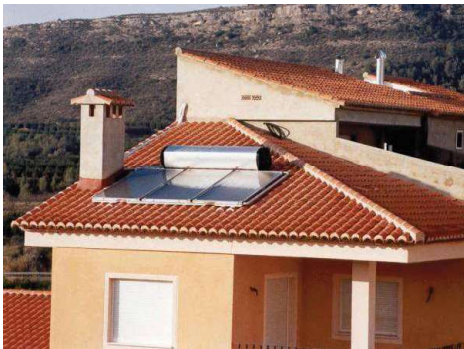
Figure 26a. Type a) Domestic Solar Hot Water System on the roof of a building (Photo: Solahart/ESTIF 2016)
