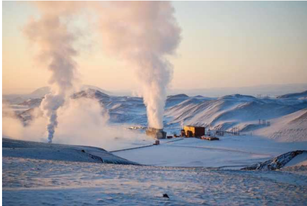
Figure 22a. Geothermal energy plant in Krafla, Northeast Iceland (Photo: David Ostman 2017)
