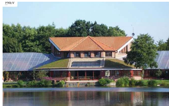
Figure 34b. Historic-Ecological Education Center Papenburg/Germany, built in 1988: Towards the North there are earth walls as energetic protection, towards the south a winter garden, which serves as semi-tropical greenhouse and as corridor between the accommodation units and common facilities. The bricks which store the temperature have been recycled. (Photo: http43 )
