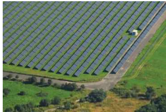
Figure 25c. Type b) Waldpolenz solarpark (40MW), Leipzig (DE). This PV system is a typical example of a large scale PV; it is built on a former military area. The modules are arranged in a parallel stripes pattern, are E-W oriented, and face the South with an optimal tilt inclination of about 30°. (Photo: Juwi Solar GmbH)
