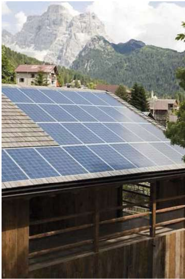
Figure 25a. Type a) Roof integrated photovoltaics, Tabià in Selva di Cadore (IT), designed by Exit. Special BIPV opaque components (modules + framing system) replace the traditional wooden tiles of the roof. (Photo: courtesy of Exit)
