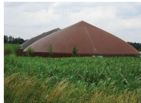
Figure 19c. Bigger biogas plant on a farm in Oberscheid, Germany (Photo: Alexandra Kruse 2016)
