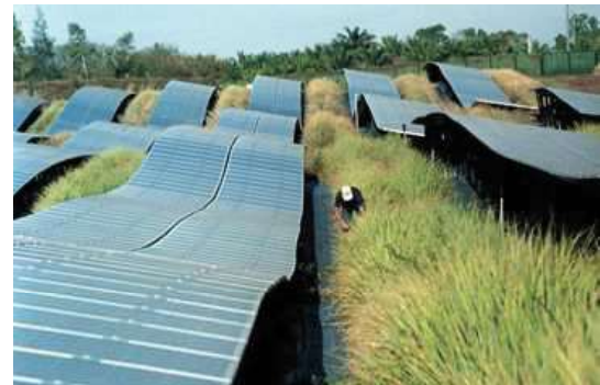
Figure 25d. Type b) Agrinergie® (2.1 MWp), La Reunion (FR). It combines energy generation from PV and lemon grass production. This dual land use design pattern enabled the developers to get the approval for the realization of a system, since in French overseas islands it is not allowed to build on ground PV, because of land and landscape protection rules. (Photo: Akuo Energy)
