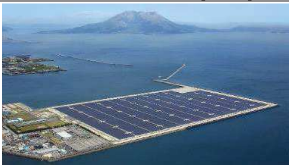
Figure 30a. The ‘Floating’ solar power plant in Kagoshima Bay, Japan can be considered as a good example for saving space. The panels over water have a cooler temperature which makes them more efficient. Finally the blue colour of the panels matches with the blue of the water, hence the panels do not disturb aesthetically. (Photo: © KYOCERA Corporation)
