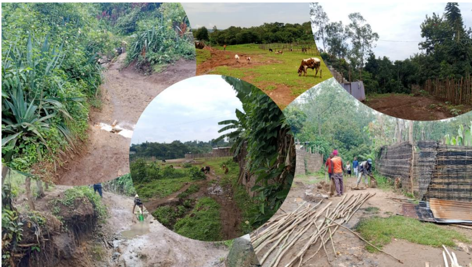
Figure 4: Critical infrastructure condition in Dilla city expansion area
