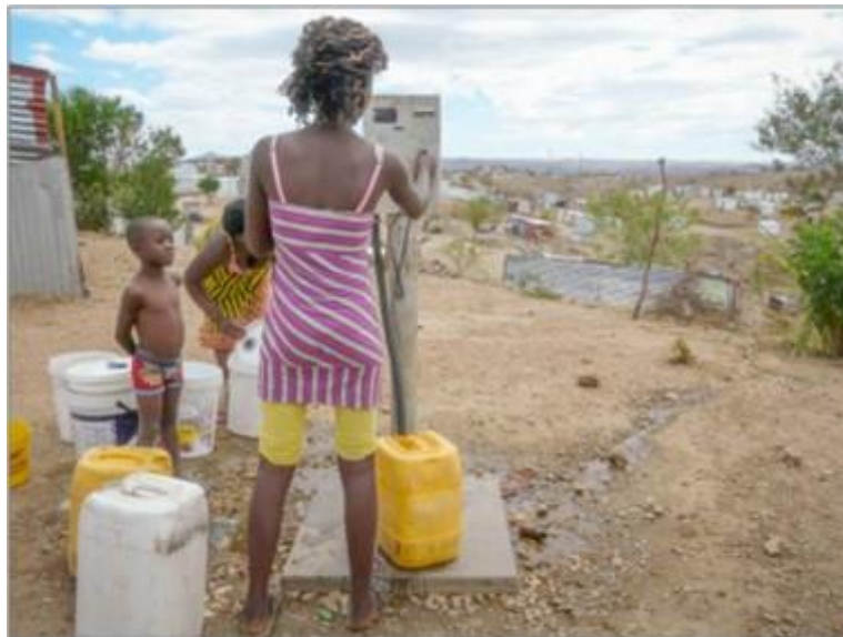
Figure 10. A prepaid standpipe water points in an informal settlement of Windhoek.
