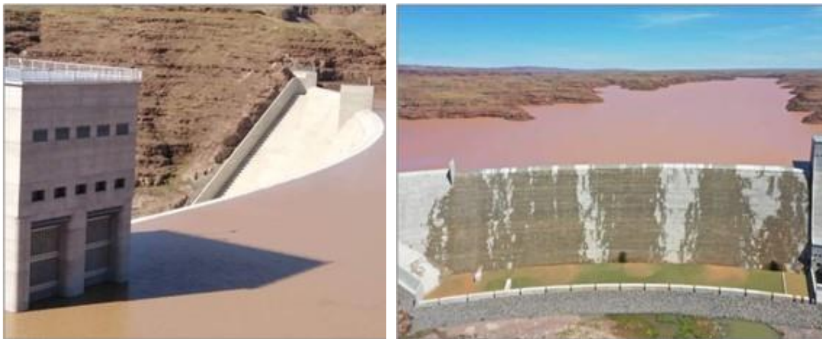
Figure 11. The first time that the newly built Neckartal dam overflowed, on 19 January 2021. It is the largest dam in Namibia.
