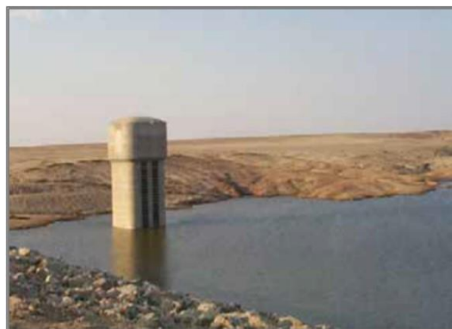
Figure 7. Omdel Dam's abstraction tower.
