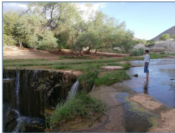
Figure 8. A sand dam at Khowarib in the Kunene Region. Source: M Coetzee.
