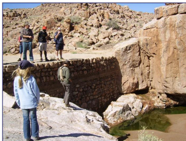
Figure 9. A sand dam on the edge of the Namib Desert. Source: M Coetzee.
