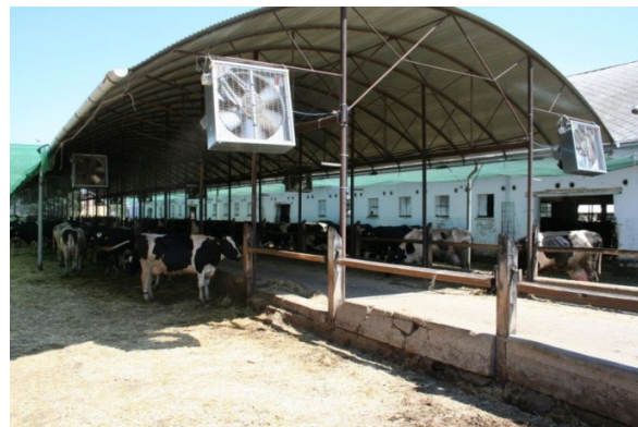
Photograph 7-8: Mechanical ventilation in freestall dairy barns with fans – Dózsa Mg. Zrt., Tass (left) és Mg. Zrt., Fábiánsebestyén (right)
