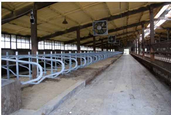
Photograph 7-8: Mechanical ventilation in freestall dairy barns with fans – Dózsa Mg. Zrt., Tass (left) és Mg. Zrt., Fábiánsebestyén (right)
