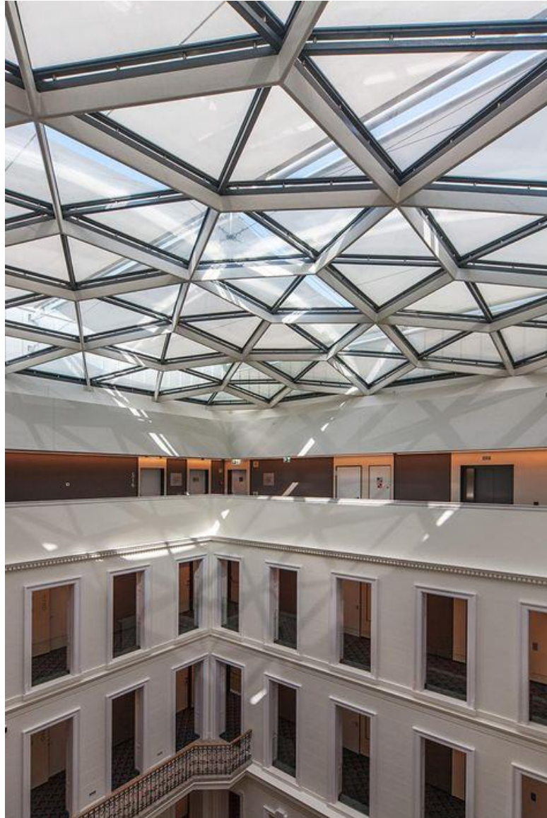
Image 2: Automatically operating shading system on top of the lobby of Hotel Moments in Budapest
