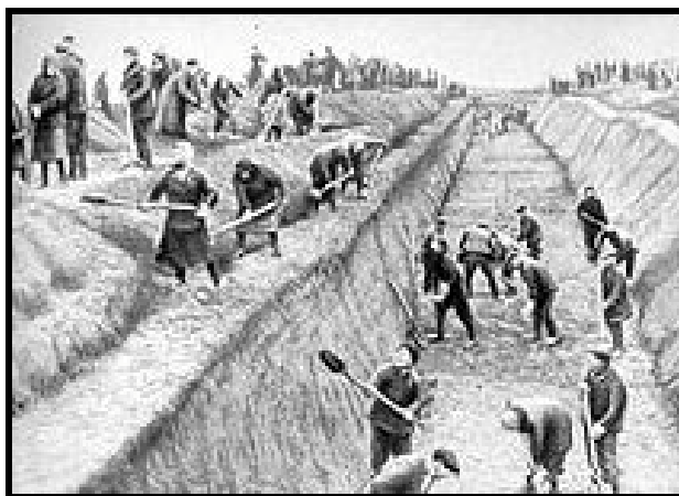
Figure 3: Building of an anti-tank dike
