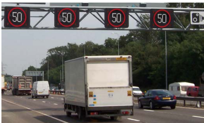
Figure 3. Variable speed limit
