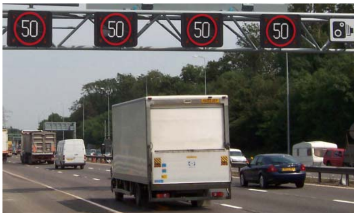
Figure 3. Variable speed limit
