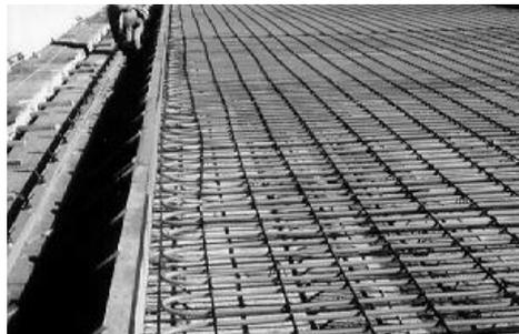
Figure 7. Heating tubes in the road surface
